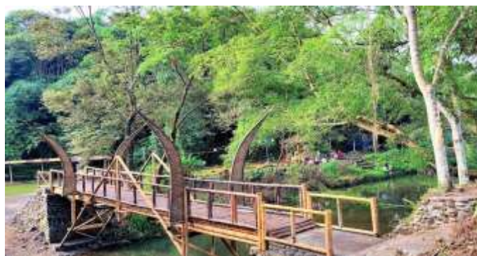
Figure 2. Natural bamboo bridge in Kedung Aren village
